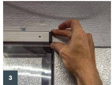
3 Secure strips with end caps.
